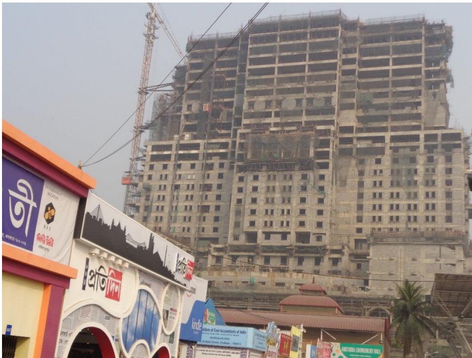
Photo 2.2 by author, 2016: ITC Sonar Hotel under construction
