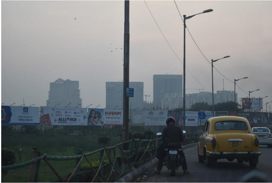
Photo 2.1, by author, 2016: New constructions along Eastern Metropolitan Bypass
