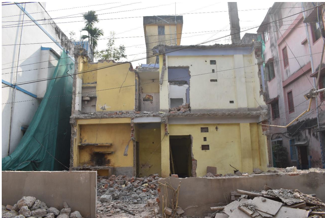
Photo 3.9, by author: A former two-storied house being demolished to pave the way for multiplex apartments
