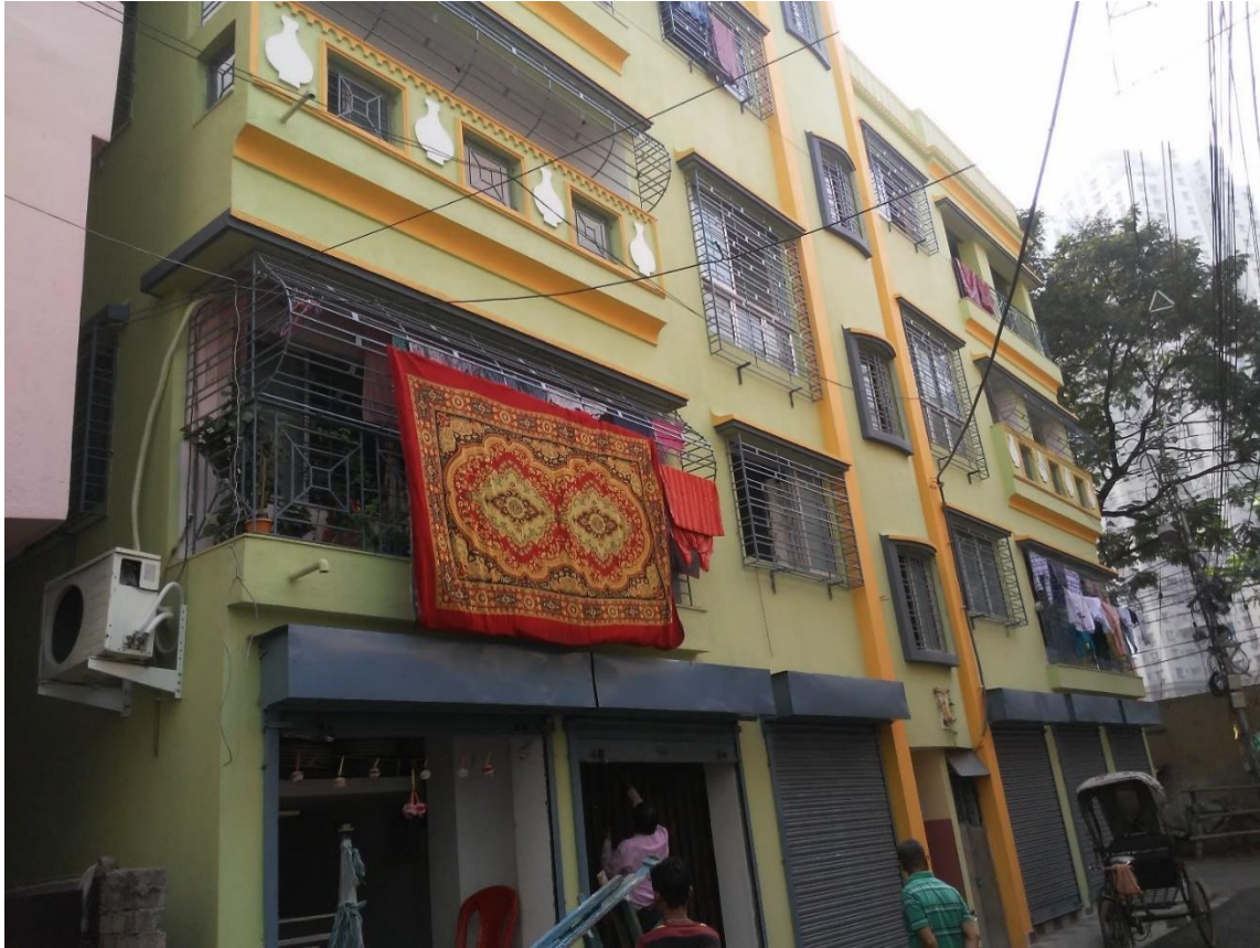
Photo 3.7, by author: A typical three-storied promoted building in Poddar Nagar
