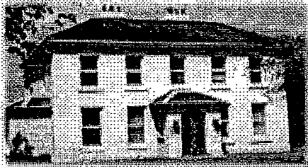
The National Technological Park's headquarters at Park House
