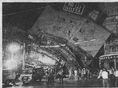
Terremoto en Taiwan. Earthquake in Taiwan, 1999
