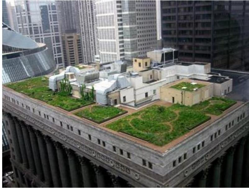
Chicago City Hall green roof,
